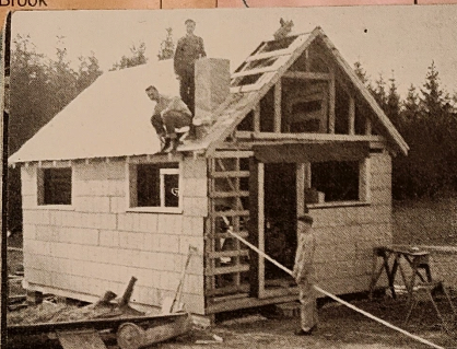
SHOP CLASS ERECTING NEW SHOP BUILDING
